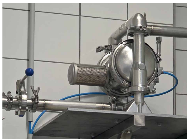
FLUX SD20 compressed air diaphragm pump in the Hygienic Design
