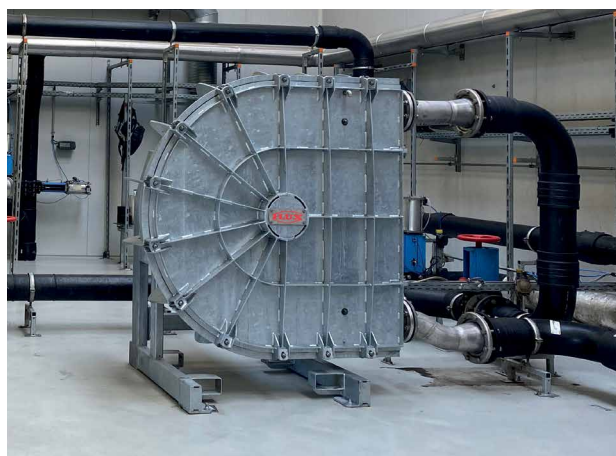
Pumping wastewater containing solids: the FLUX-FHP achieves displacement volumes of up to 300 m 3 /h.
